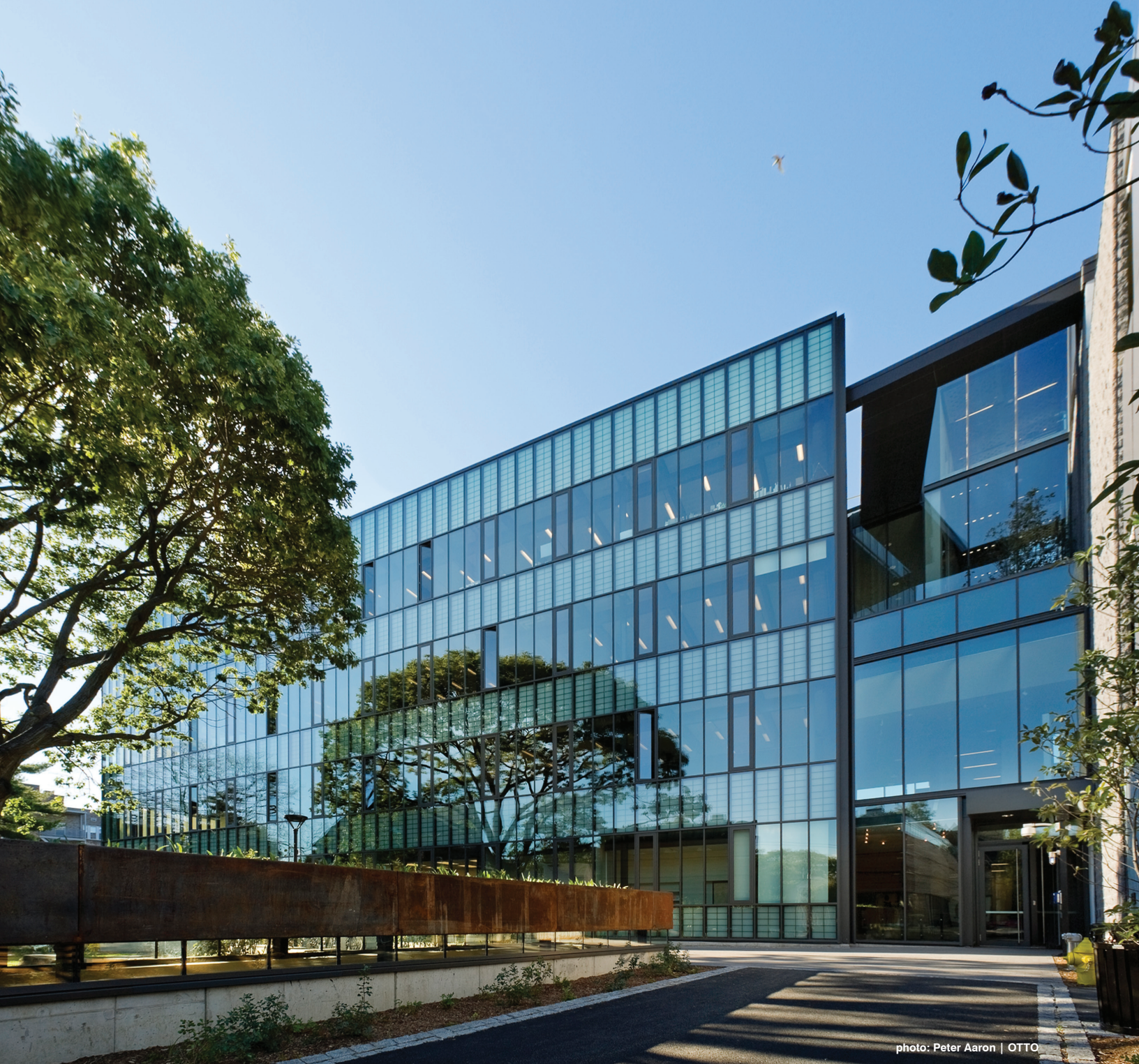
Yale Sculpture Building | New Haven, CT | Kieran Timberlake Architects | Double Skin Facade System with Schuco® and Kalwall+Lumira (above)
