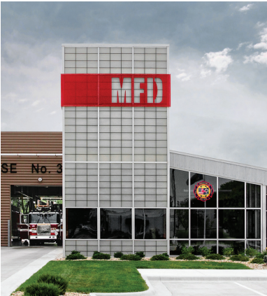
Manhattan Fire Station | Manhattan, KS
