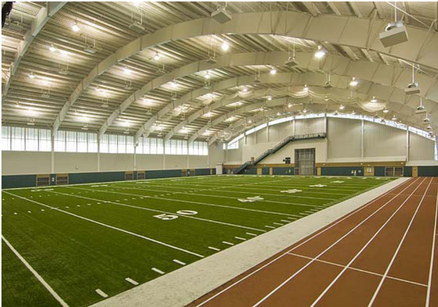
Colorado State University Football: Indoor Practice Facility Ft. Collins, CO | Aller Lingle Massey Architects
