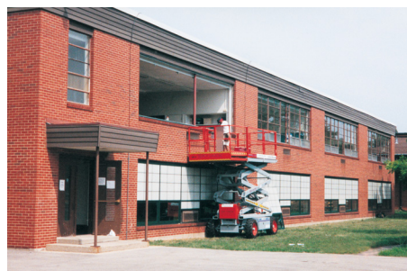
During Window Replacement
