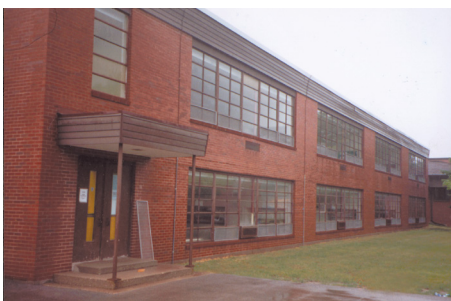
Before Window Replacement
