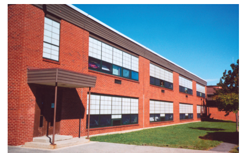
After Window Replacement
